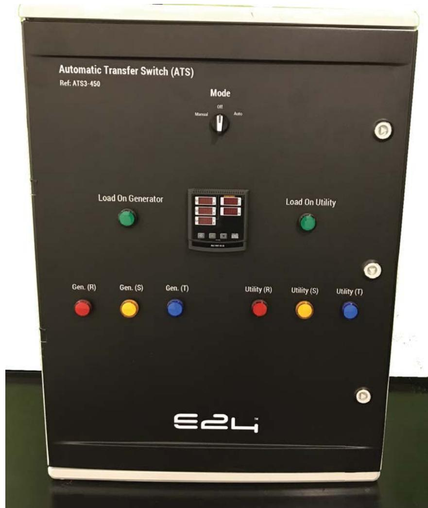
Automatic Transfer Switch Panels (ATS) are mainly electrical switches that switch the load between two sources. It is used when the client has a backup diesel generator and wants to integrate it with E24's Energy Storage System (ESS). ATSs supplies the input of the ESS and switches it between utility and diesel generator.
